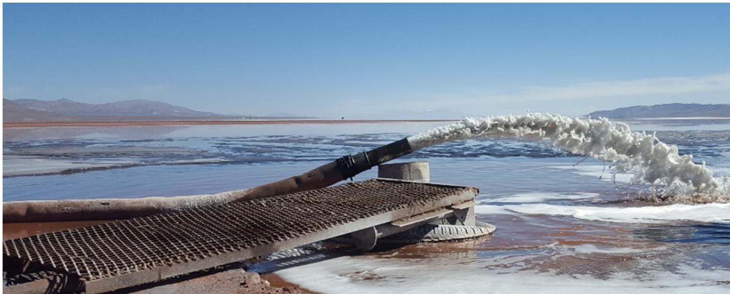
Figure 3: Pumping from sand units in CAU11 at Cauchari
